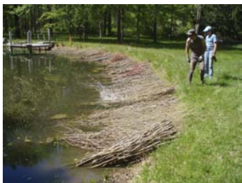
Willows harvested in March, taken out of cold storage days prior to use and allowed to "soak" in nearby pond.
